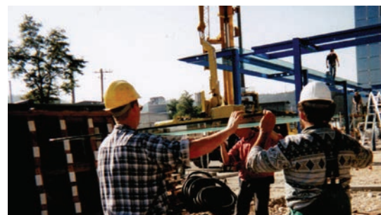
Work on the construction site
