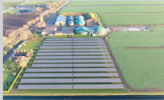
2 MW Nieuweroord Solar Park The Netherlands 2018
