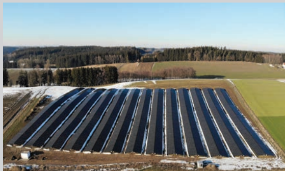
3 MW Aiching Solar Park Germany 2018
